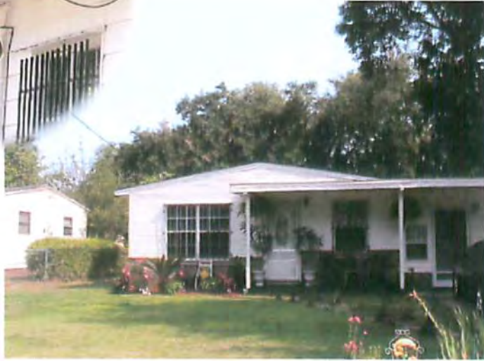
Roof replacement – 1125 Medford Drive
