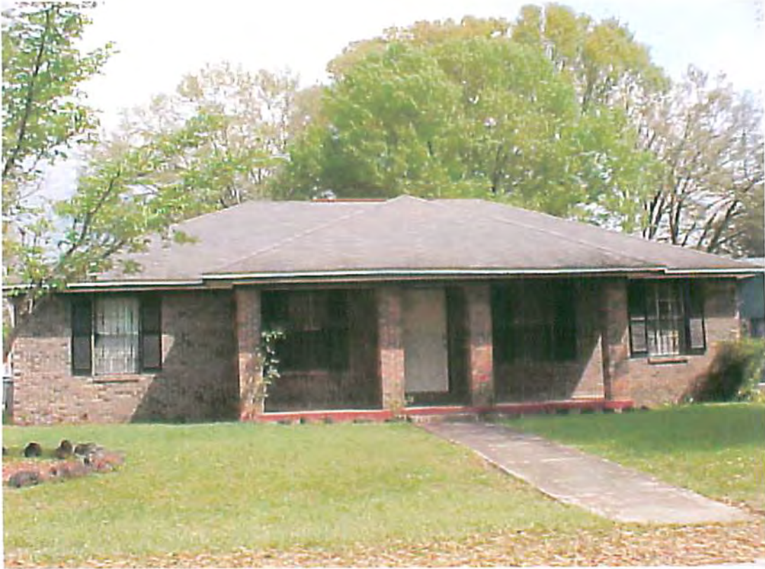
ROOF REPLACEMENT – 2324 AVERY STREET
